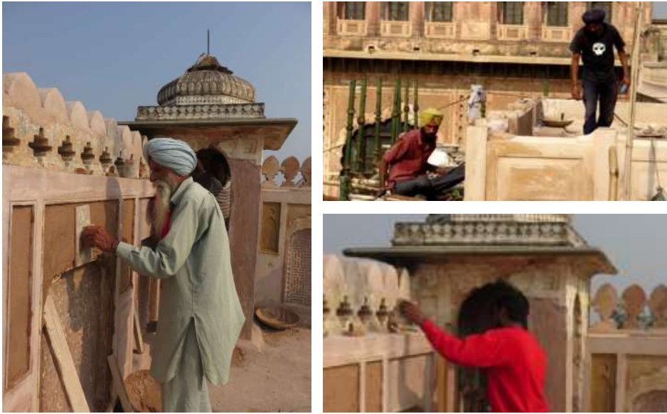
Figure 13. Intergenerational workshop to share traditional building techniques © Abha Narain Lambah Associates, 2013.
